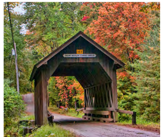
Figure 1-6 Swamp Meadow Covered Bridge
